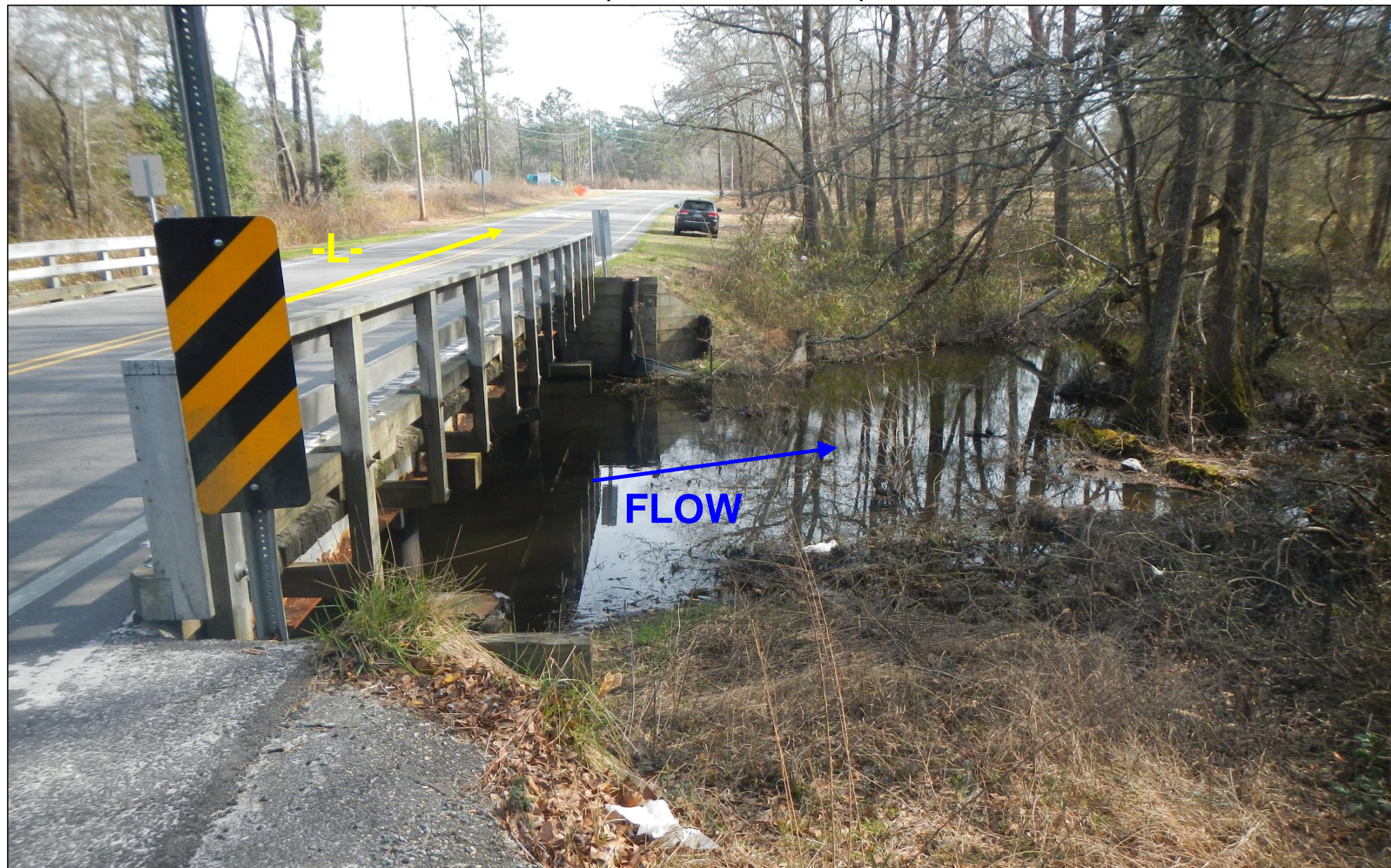
Looking Upstation from Sta. 16+75, -L-
